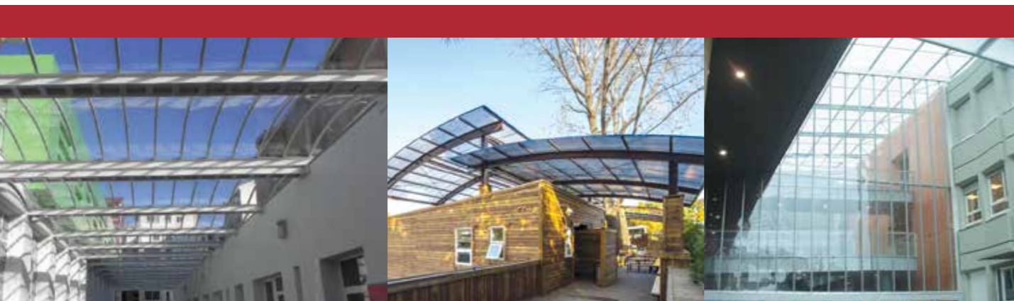
Zankoeta School, Spain Danpal® Compact Architect: José Montajes Mentxaka
