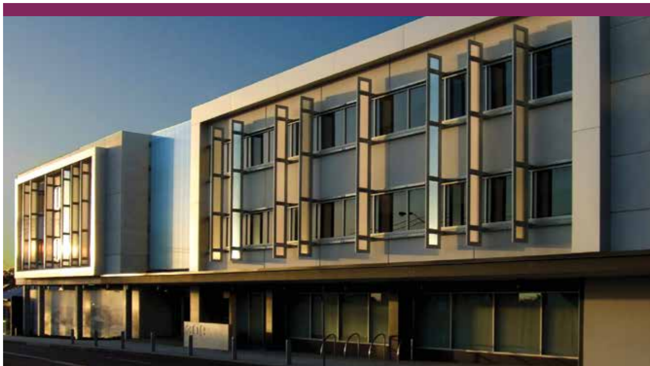
Community Services Offices, Charlestown Australia | Danpal® Louvre System | Architects: Jackson Teece
